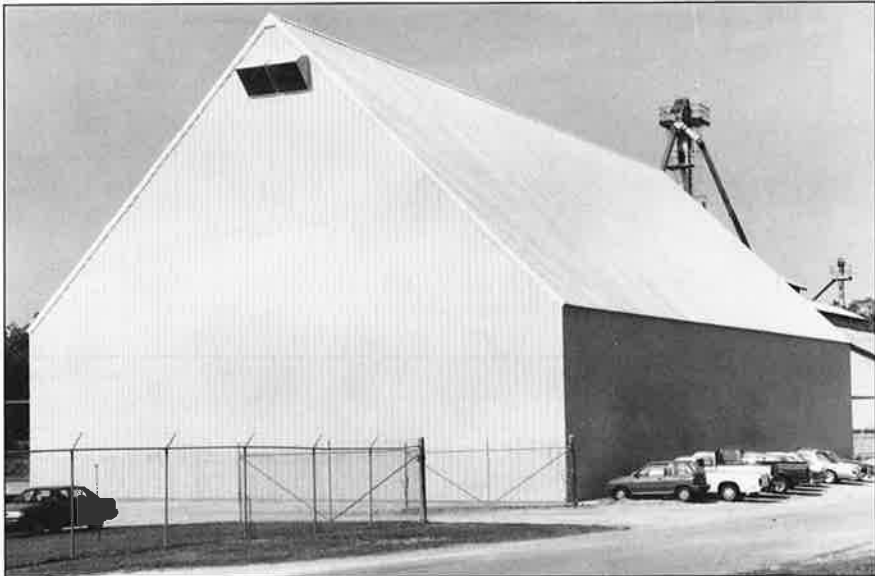
Fig. 1. Mechanically ventilated conventional flat-type storage warehouse for farmers stock peanuts with a 45 degree roof slope (12/12).
