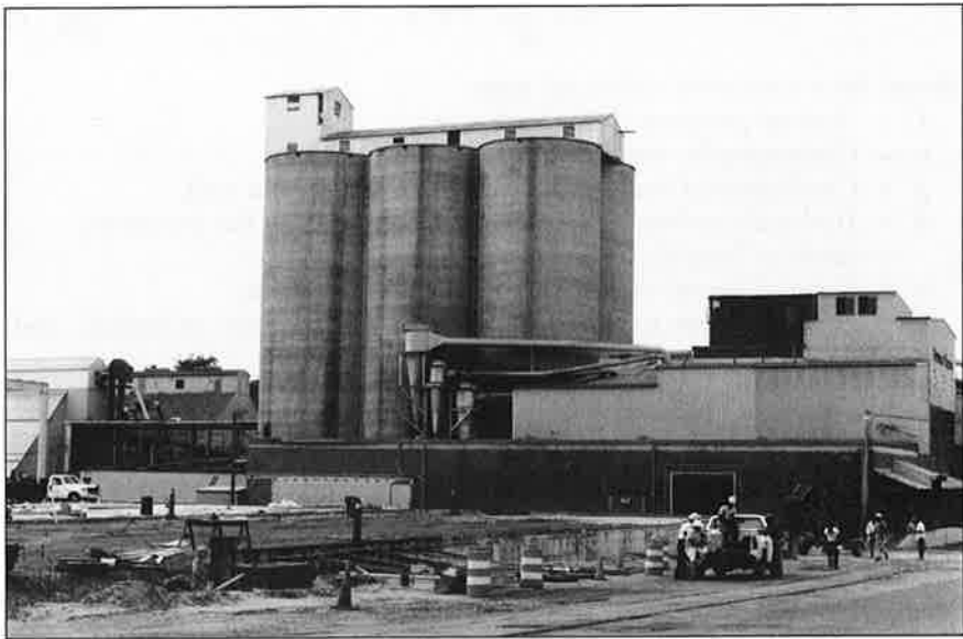
Fig. 5. Concrete silos used to store farmers stock peanuts.
