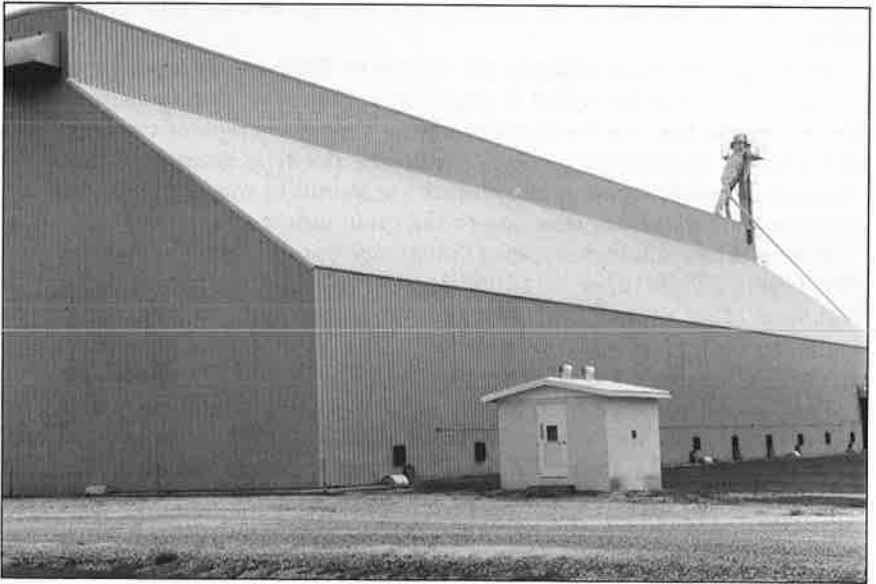
Fig. 2. Conventional flat-type storage warehouse for farmers stock with “doghouse” structure on top and a 37 degree roof slope (9/12).
